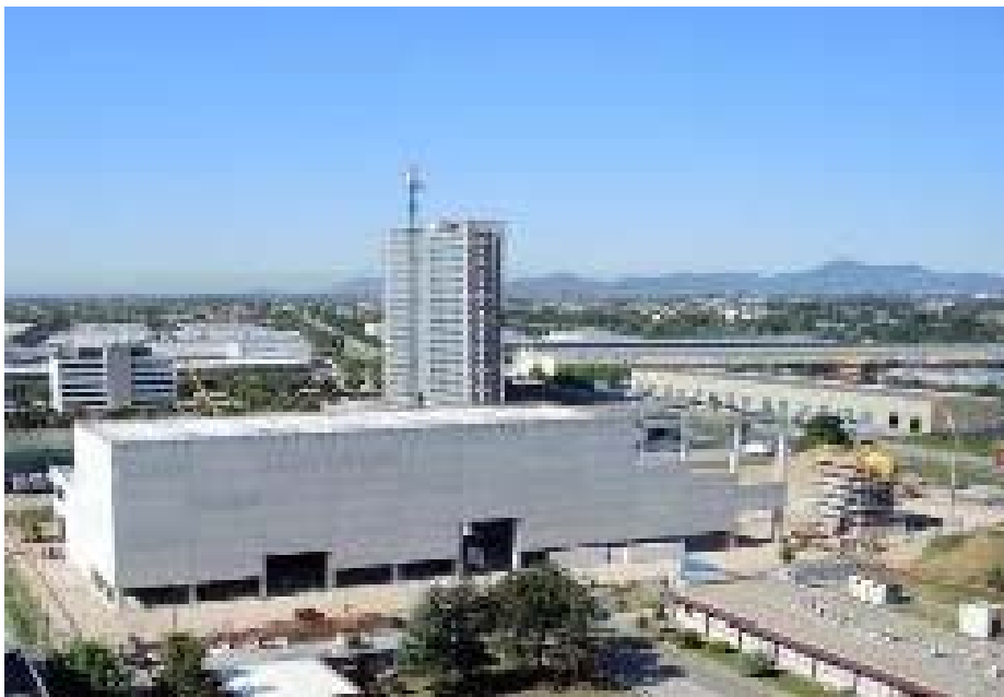
Neutral Beam Injection System
